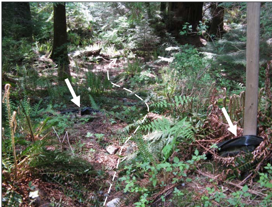
Photo 24. Abandoned silt fencing (arrows) along stormwater discharge route within Terminal Creek ravine. Dashed arrow denotes stormwater route when flow is present. This site is within the IPS property immediately east of Belterra lands. 19-Jun-09
