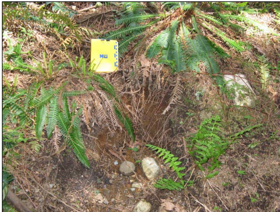
Photo 30. Minor erosion of Terminal Creek ravine bank below IPS parking lot stormwater discharge. Note exposed roots. 19-Jun-09
