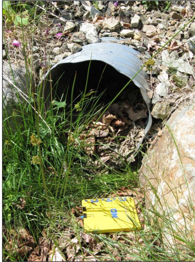
Photo 21. Outlet of upper culvert on Belterra driveway. Discharge from this culvert ultimately discharges to Terminal Creek ravine near east boundary of the property. 19-Jun-09
