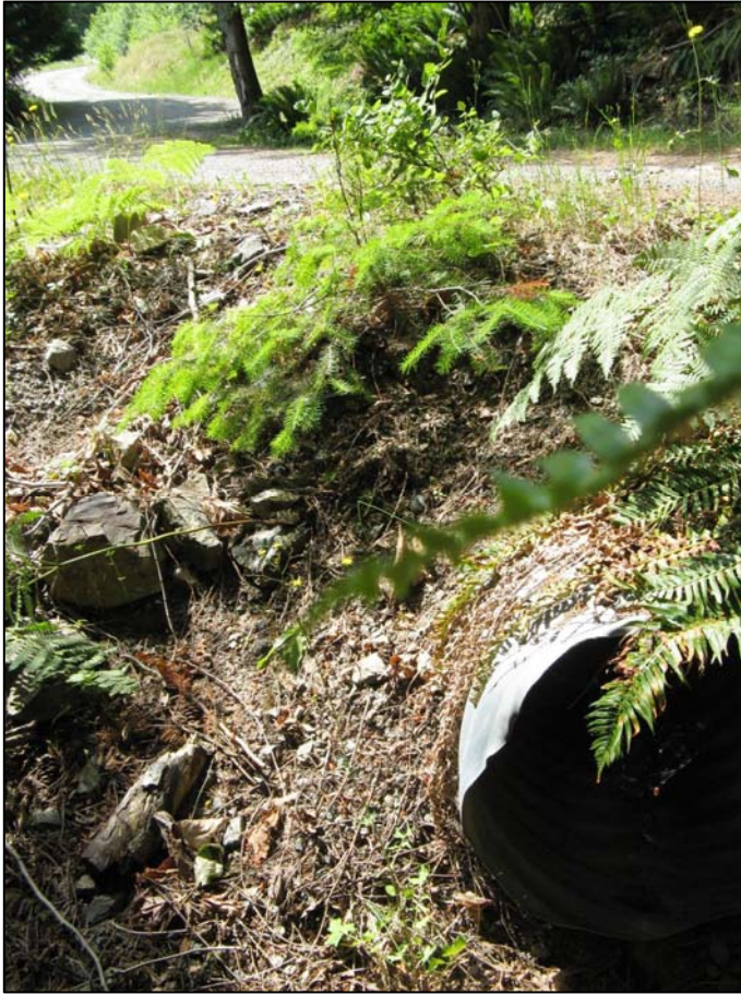
Photo 27. Outlet of culvert under Carter Road, viewed toward Belterra driveway. This culvert carries all drainage from the lower and eastern half of the Belterra lands. 19-Jun-09
