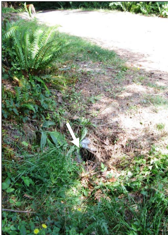
Photo 26. Culvert (arrow) under carter Road at bottom of Belterra driveway, viewed to north. Note accumulated vegetation and leafy debris at culvert inlet. 19-Jun-09
